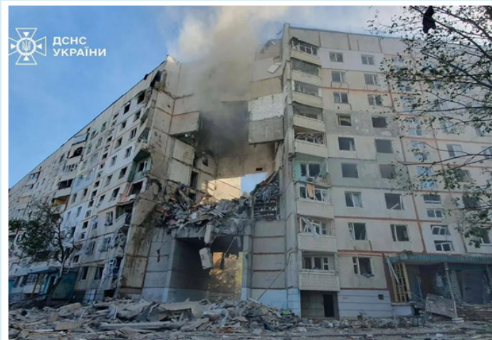
Figure 2: The collapse of the structures of a residential building in the city of Kharkiv due to the impact of a Russian ballistic missile, where the residents remained injured.
