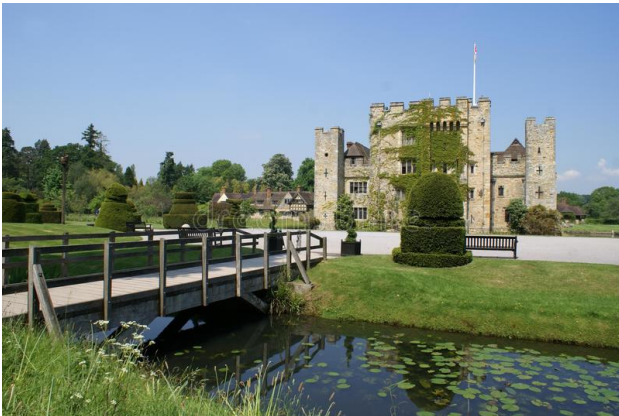
Fig. 59. The bridge over the River Eden. running in front of Hever Castle garden in Hever.
