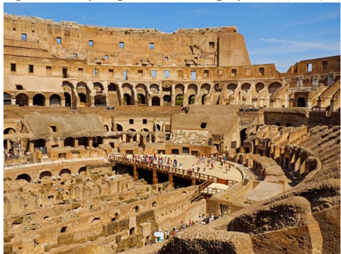
Fig. 8. Interior of the Colosseum.
