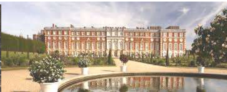
Fig. 25. Hampton Court Palace. Architectural style Baroque.
